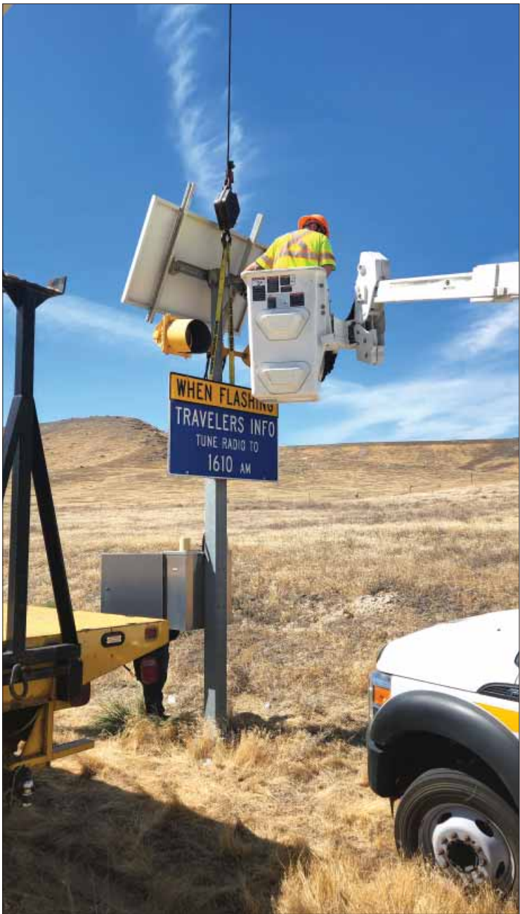
An ITD worker installs a solar panel on top of a reclaimed federal highway communication sign to recreate an open range warning sign. Submitted photo
