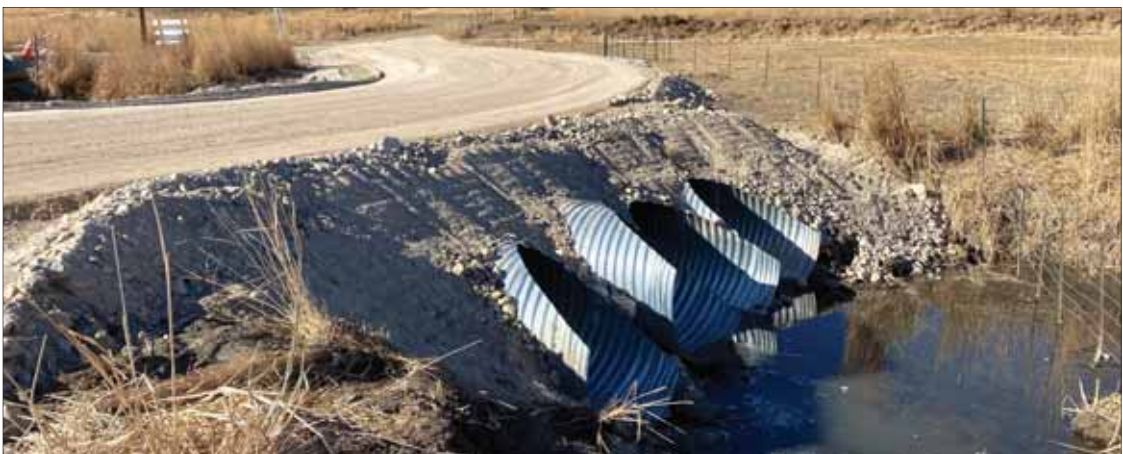
The Idaho Transportation Department has completed the temporary Salmon Creek Road bypass. Submitted photo
