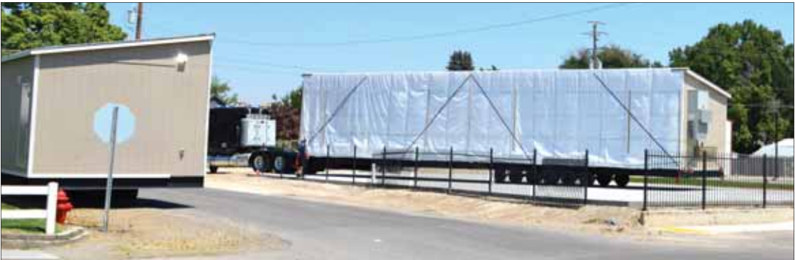
The first half of a new modular classroom was put into place near the Trojan Tots pre-kindergarten building on July 16.
