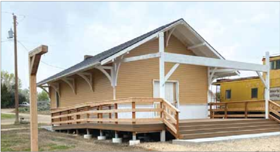
The Marsing Depot has been restored to its original paint scheme, and a new stage awaits the Outpost Days musical offerings. Submitted photo
