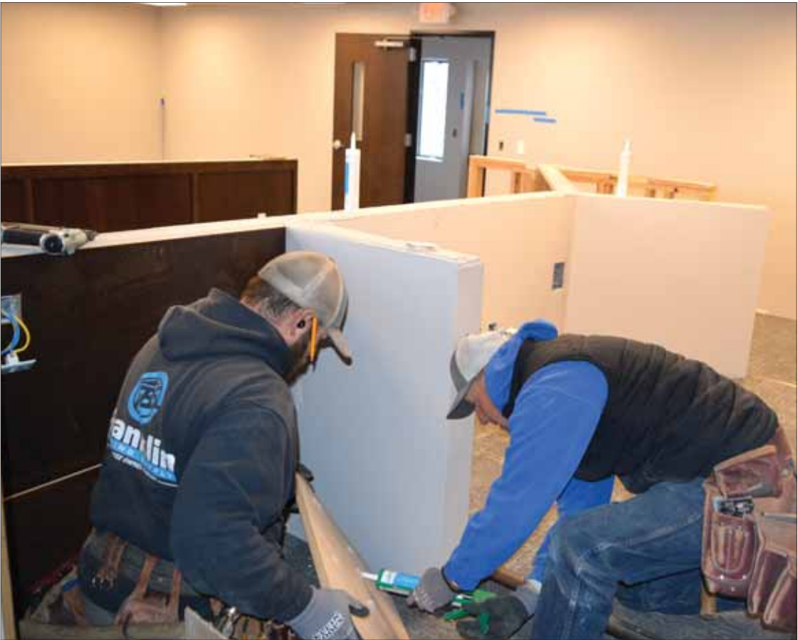
Dusty Darbin (left) and Aaron Marts work to apply dark trim facade to the bench in the new magistrate courtroom in Homedale.
