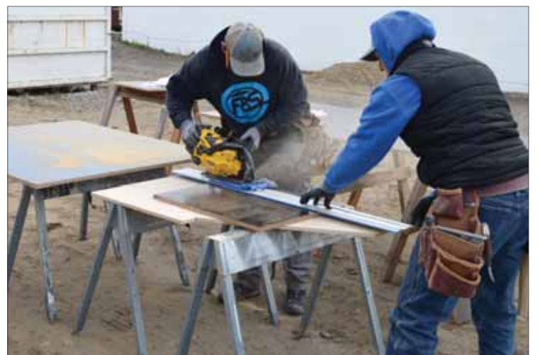
Dusty Darbin (left) cuts trim for the courtroom as Aaron Marts holds the straight edge last Wednesday.
