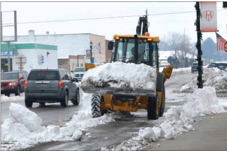
Homedale Public Works acting supervisor Kurtis Stansell removes snow that had been covering a storm drain on East Idaho Avenue on Friday.
