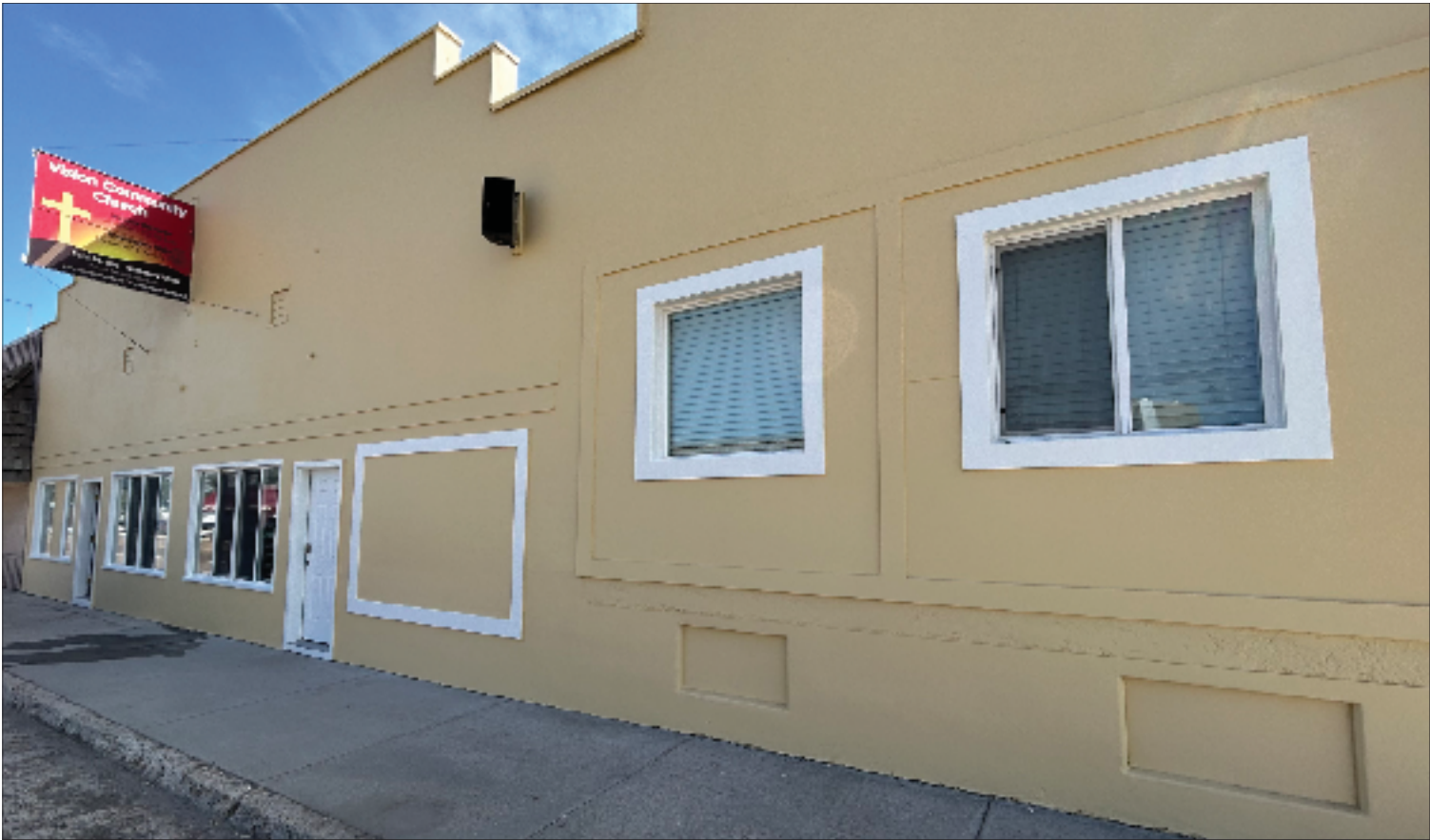
Vision Community Church on Main Street was the first recipient of the Marsing Beautification Project's plan to spruce up storefronts throughout downtown. Left: New paint and trim brightened the portion of the building facing Main Street. Below: The building as it looked before project volunteers swarmed into action. Submitted photos
