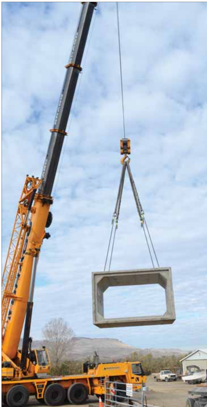
Above: A crane operator swings a box culvert toward South Canal on Johnstone Road on Thursday. Bottom: The crane operator was able to steady the cement box so other workers could place the culvert next to its neighbor.
