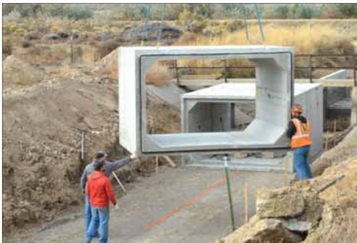
Above: A crane operator swings a box culvert toward South Canal on Johnstone Road on Thursday. Bottom: The crane operator was able to steady the cement box so other workers could place the culvert next to its neighbor.
