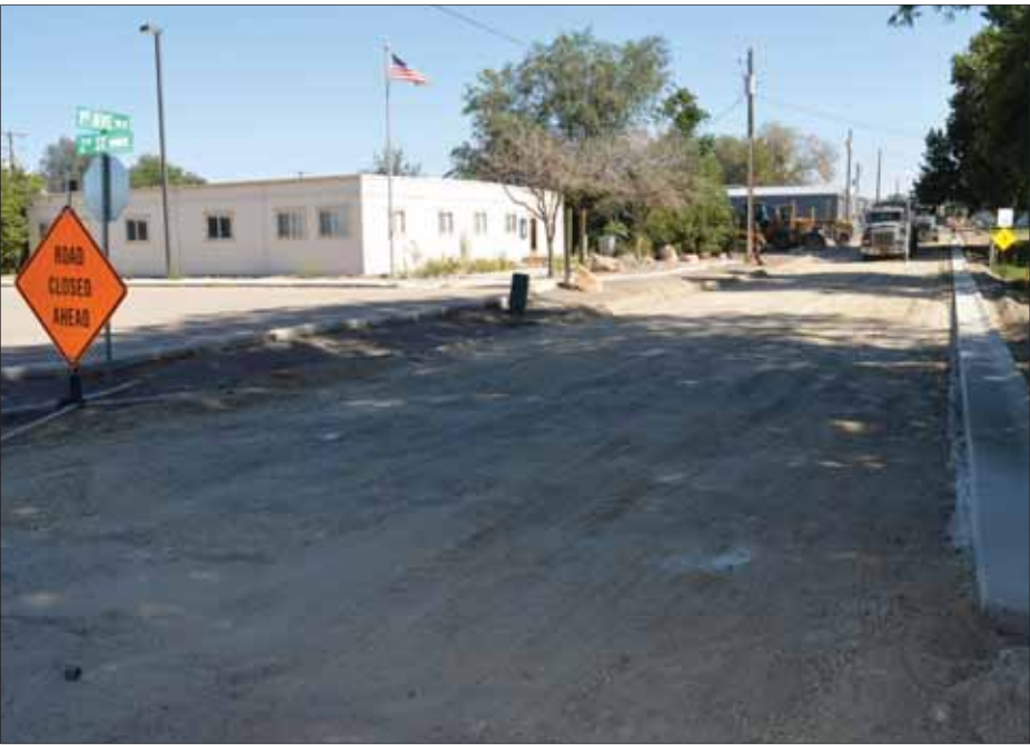
After building curbing and gutters, a construction crew worked last Wednesday to put down a road bed on 1 st Avenue West between West 2 nd Street North and Main Street. Paving was to commence Friday, but hadn’t started by the afternoon. The former Bureau of Land Management Owyhee Field Office building (left, background) is scheduled to be moved to the Marsing Labor Camp this week.
