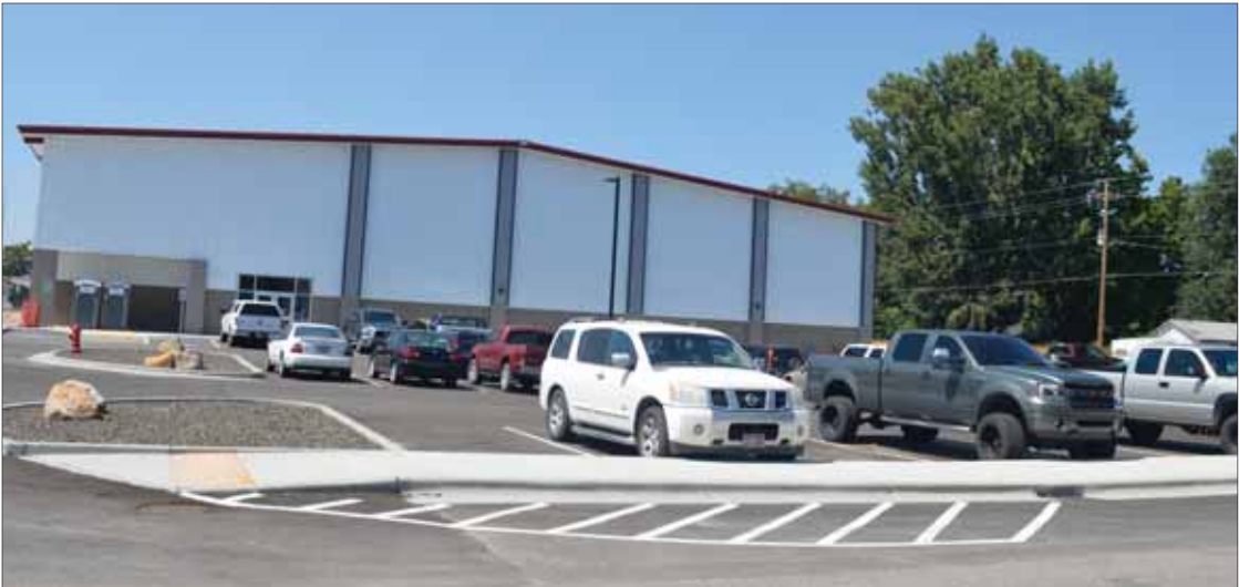
The new auxiliary gymnasium construction included sidewalk and a paved and lighted parking lot to provide more student parking during the school day. The sidewalk was extended north to ring the existing paved lot to the east of the main gym, providing more organized parking.
