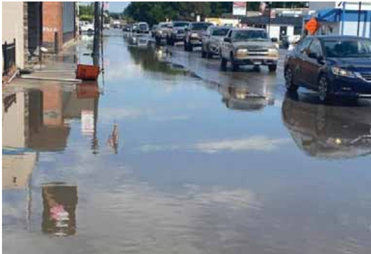
Storm drains couldn't handle the volume of rainwater, and Idaho Avenue and Main Street flooded. Photo by Joshua Gray / GrayHawk Photography
