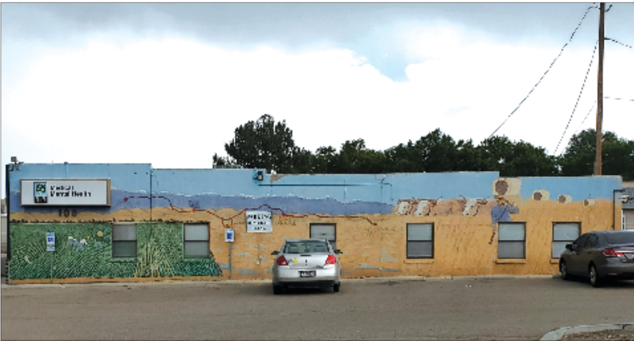
One last shot of the full mural on the Terry Reilly Health Clinic's west wall in Homedale was snapped before partial demolition began. TRHS photo
