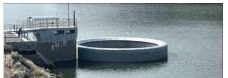
The Owyhee Reservoir water is up to the ring gate for the first time in at least three years. Owyhee Irrigation District photo
