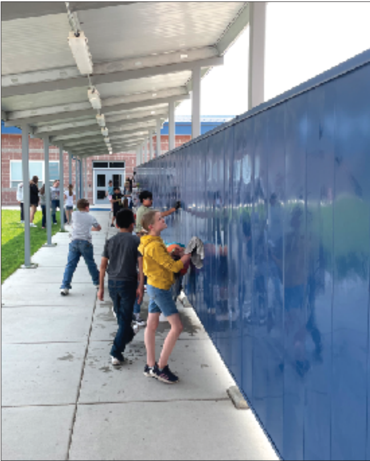
Students put a new coat of blue paint on the wall along the walkway between the elementary school and the cafeteria.
