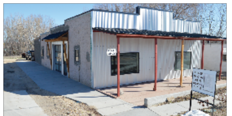
Work has already begun on the building that will be part of a proposed food truck park in Marsing.
