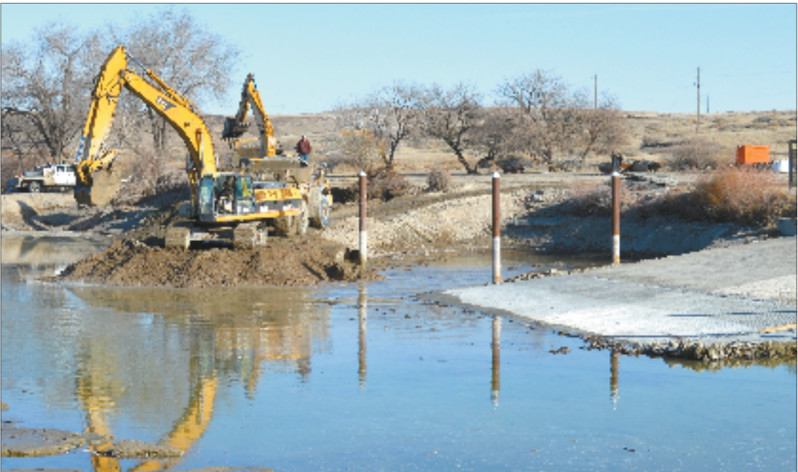
Above: Heavy equipment from Robison Logging and Excavation was on the job for the first weeks of the year dredging a deeper channel as the boat ramp cement slab (right) was extended. Below: The opening of the vault restroom last week paved the way for the reopening of the Black Sands boat ramp area. Submitted photo
