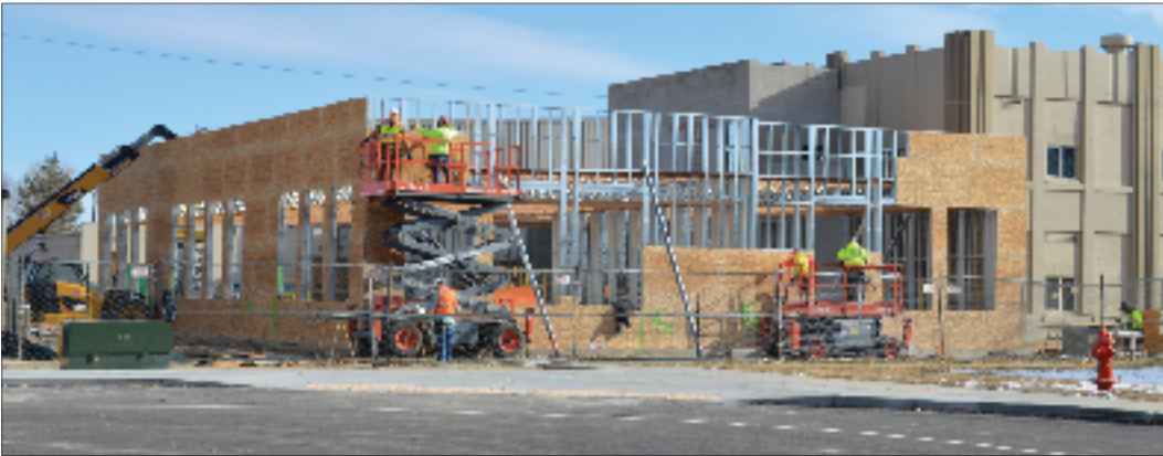
One of many construction projects started in Homedale last year was a new classroom building at the high school.
