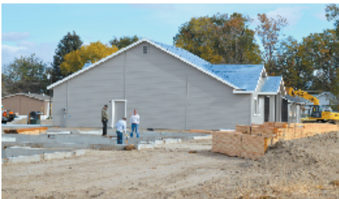
Residential construction was rampant throughout the county and especially in Homedale, such as the new homes being built a stone’s throw from the fairgrounds.
