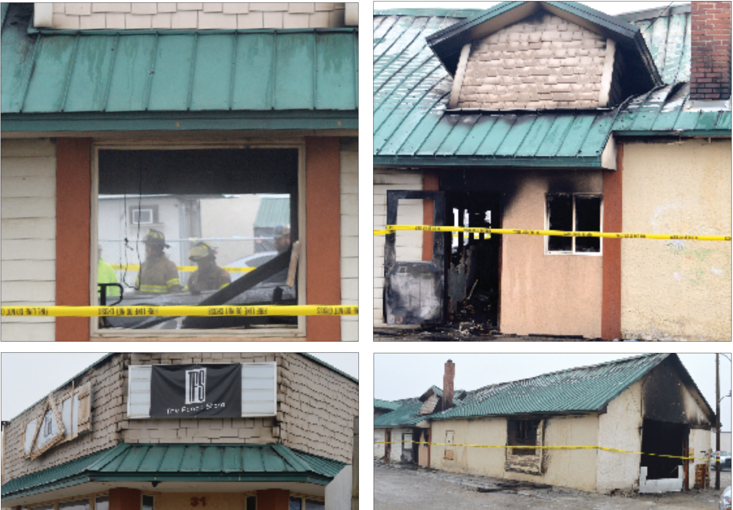
Counter-clockwise from top: A dormer collapsed and a door was scorched on the west side of the building. Firefighters inspect damage on the east side of the building. Sheetrock is piled at the entrance to The Fence Store, which was a total loss. The fire burned the length of the building, blackening every doorway and window frame.
