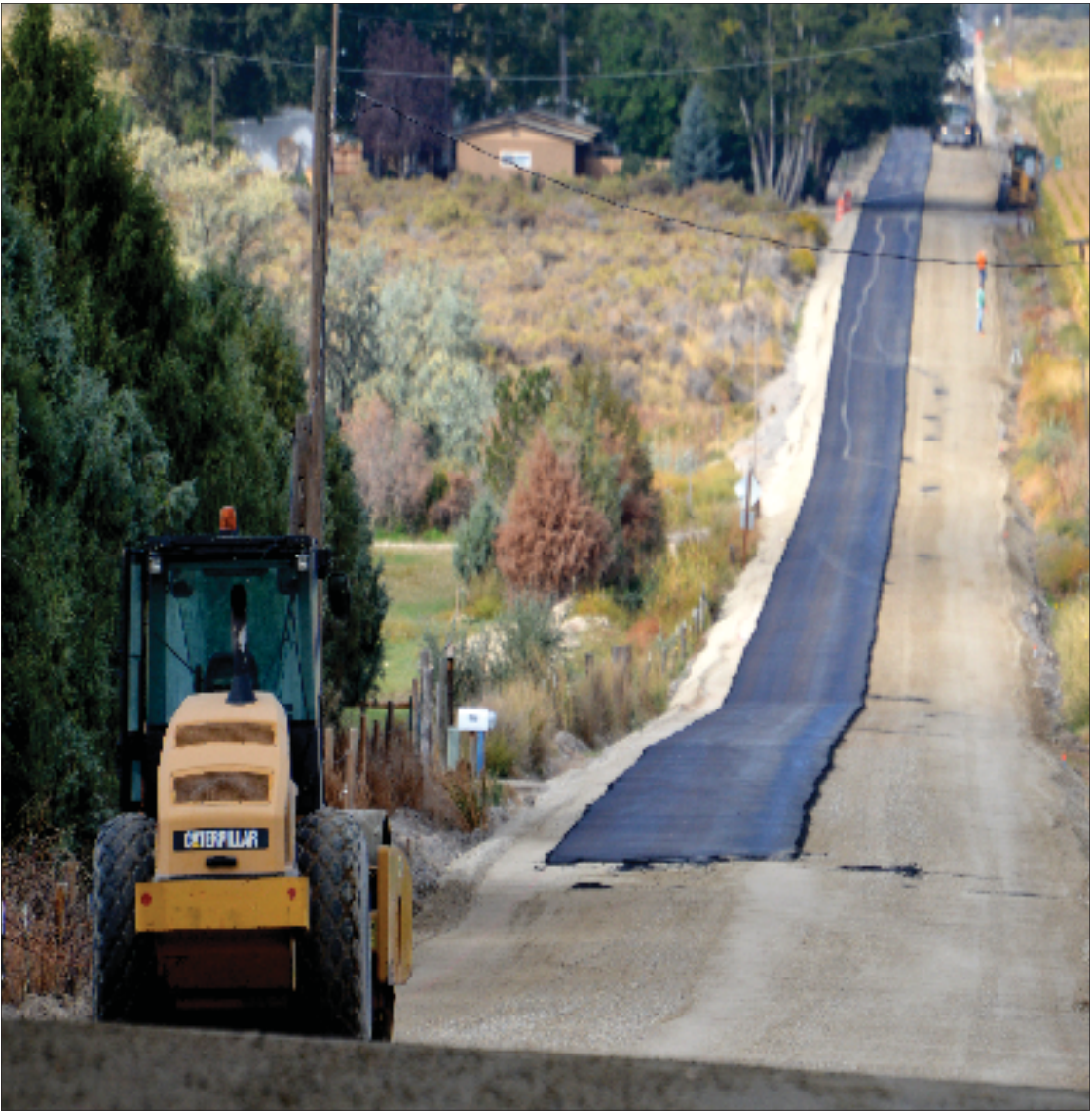
After rebuilding the roadbed to ensure proper drainage, a Showalter Construction crew put down blacktop on a long stretch of Cemetery Road between Y Road and South Jump Creek Road last week. The project was completed Friday, according to Homedale Highway District director of highways Dan Herman.
