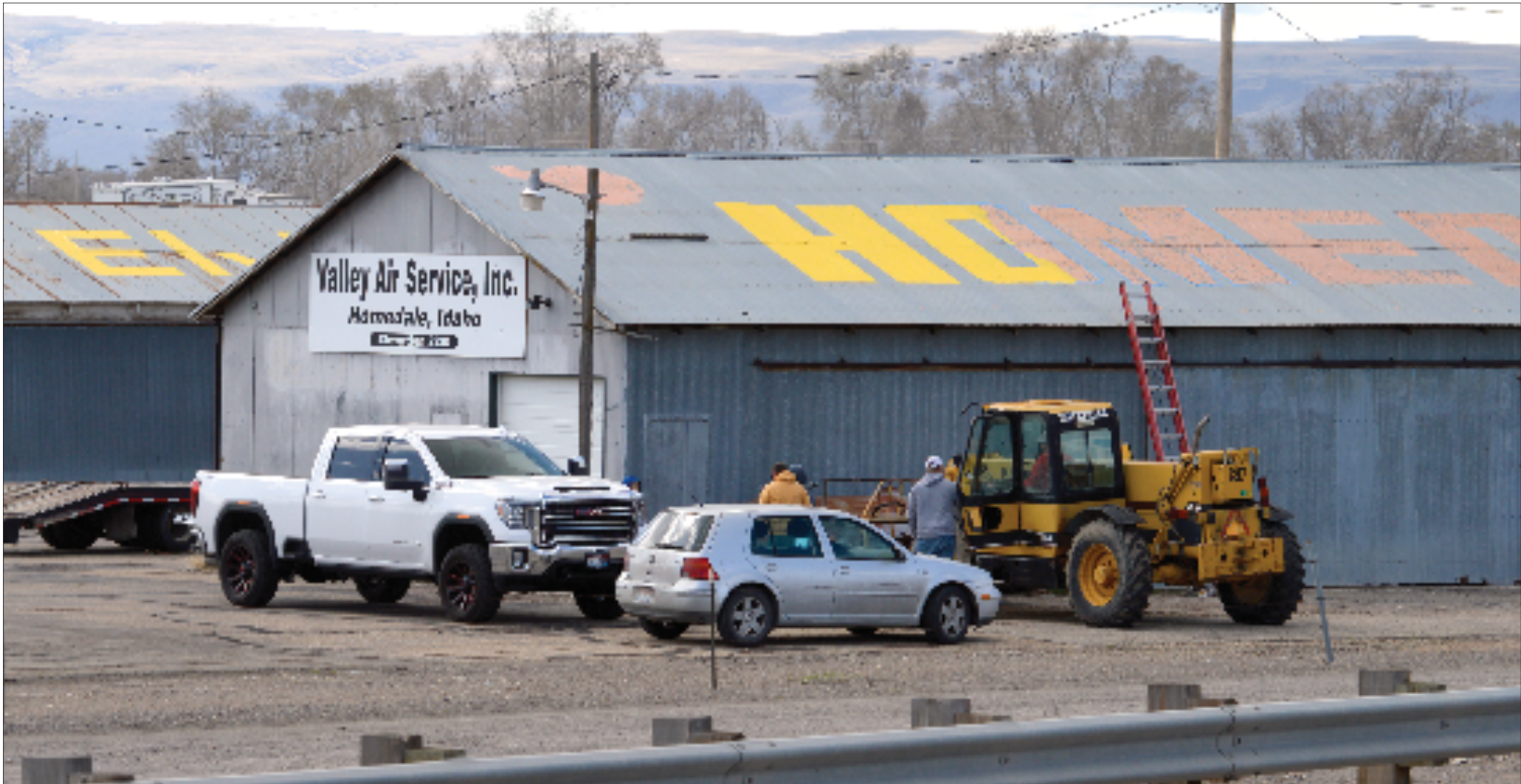
Back in April, a crew repainted the large “Homedale” sign atop the Valley Air Service hangar after earlier painting the elevation of the city municipal airport on an adjacent building. The work was part of 2022 Homedale High School graduate Eli Heck’s senior project and is the latest private upgrade at the airport. The work now will be complemented by major publicly funded upgrades at the airport, according to the Idaho Transportation Improvement Plan released by the state last week.
