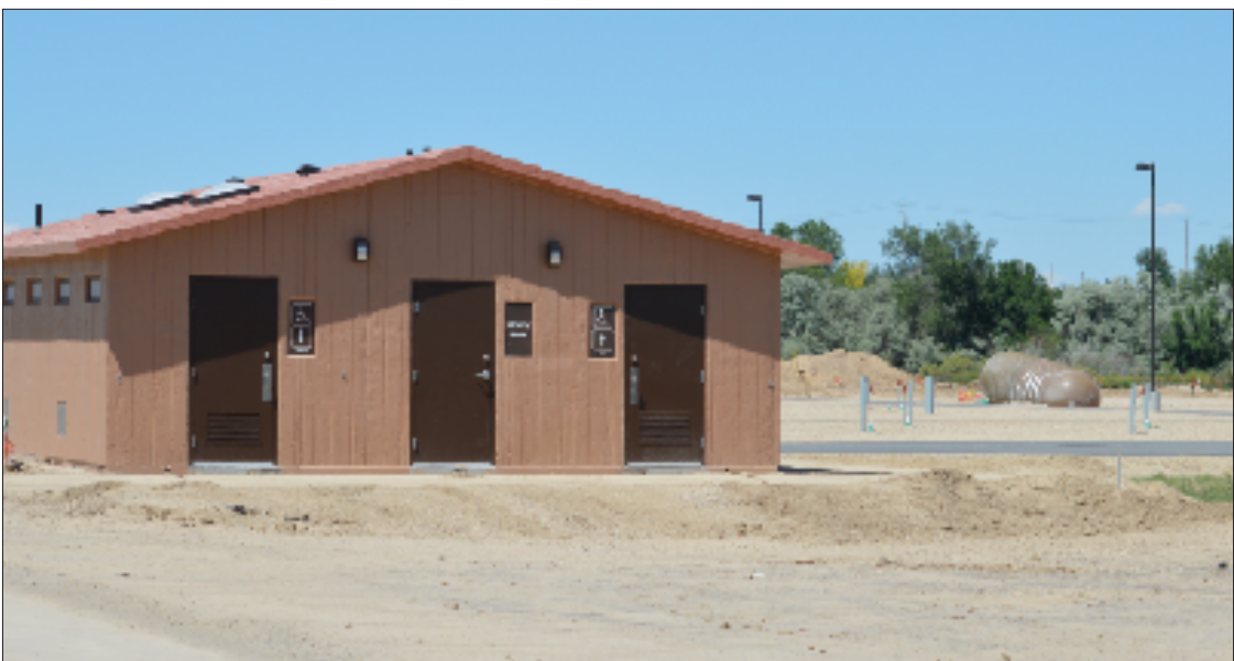
After a hiccup, the new three-piece modular restroom is in place at the Owyhee County Fairgrounds near the new paved and electrified RV park.
