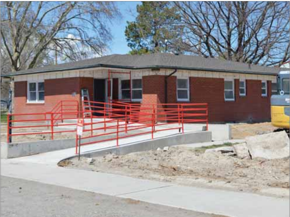
Work has been steady to convert the old St. Hubert's rectory into a preschool building, including the addition of bright red metal hand rails.
