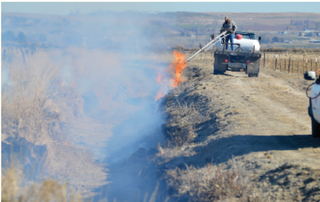
The South Board of Control maintenance crew took steps to prepare area ditches for water last month, burning weeds from the banks near Jump Creek off U.S. Highway 95.
