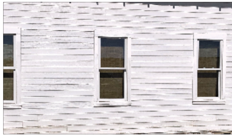
The Oreana Community Hall finally has new, more efficient windows. Submitted photo
