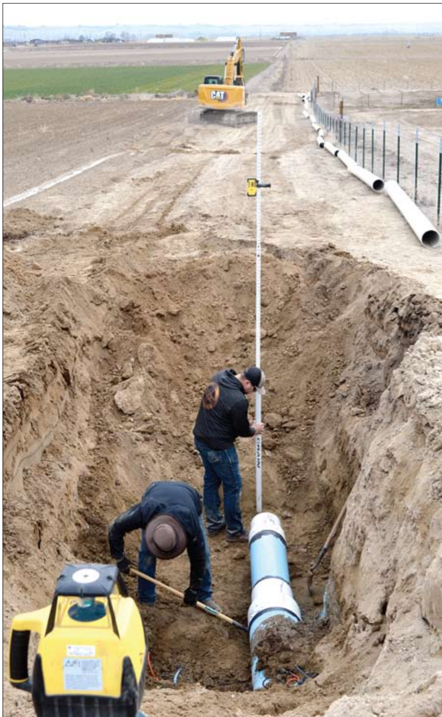
South Board of Control maintenance crewmembers Bill Maxwell (left) and Mike Boyce continue work to pipe the 4.3 lateral to provide area producers with pressurized irrigation for pivots and water conservation.
