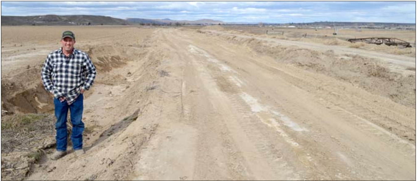
Greg Purdom stands at the edge of a settling pond that the South Board of Control helped dig to keep field run-off — and accompanying sediment — from crossing a road and draining into an irrigation ditch.
