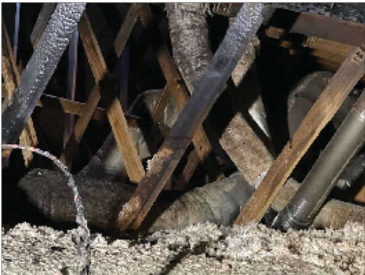
Chantell Lee said the fire started outside the home, traveled up the wall and destroyed beams and HVAC equipment in the attic. Submitted photo
