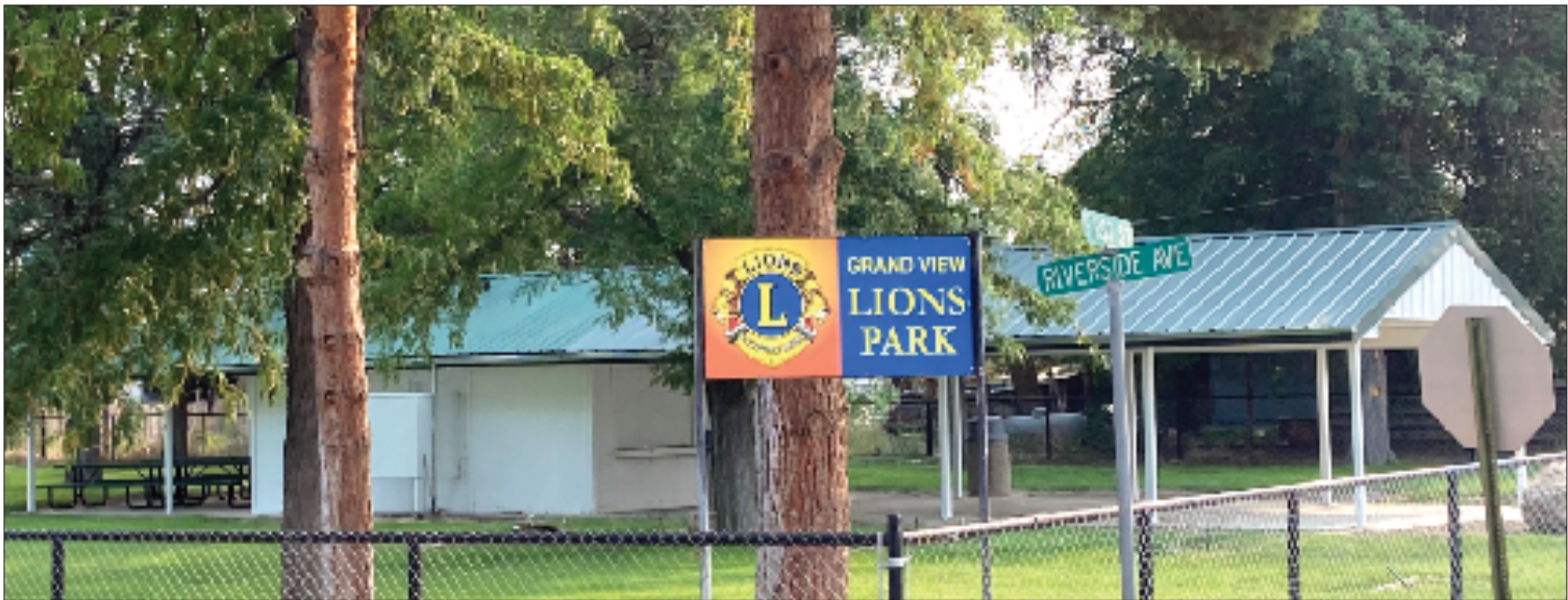
The rebuilt Lions Club hall includes a patio and outdoor kitchen on the grounds of the namesake park in Grand View. The park has new fencing, too, thanks in part to local Eagle Scouts projects. Submitted photo
