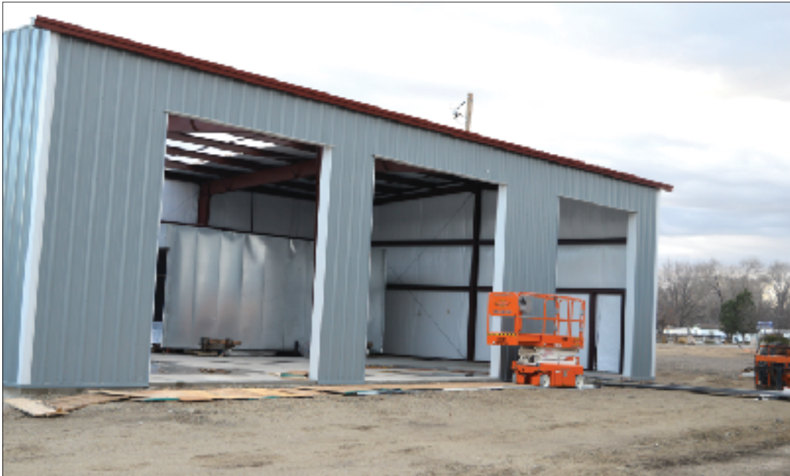
A new shop has been built directly east of a building that was part of the old Homedale Feed property.
