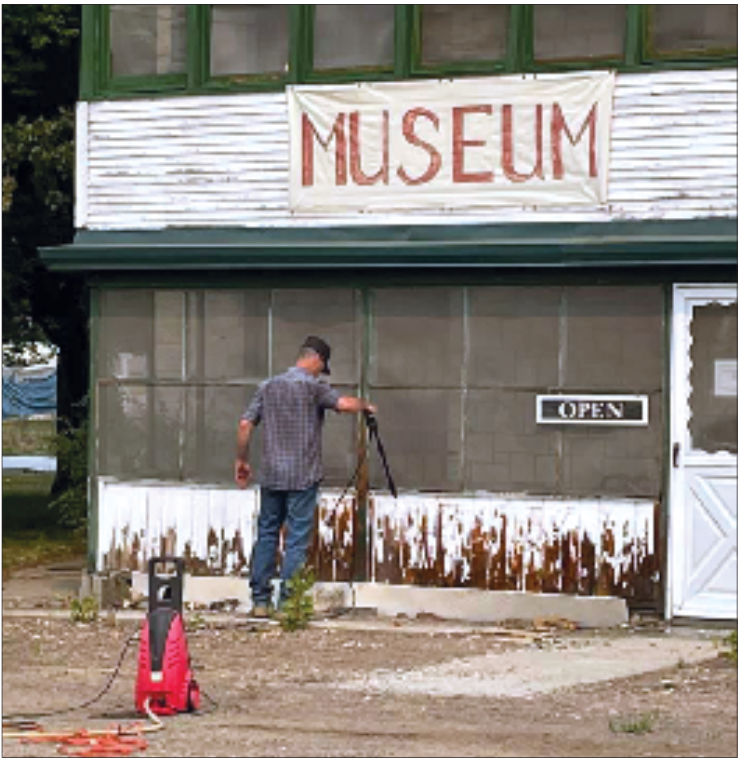
Above: The old paint is removed from the front of the Jordan Valley ION Heritage Museum in preparation for a makeover. Left: A worker affixes the new museum banner to the front of the building. Submitted photos
