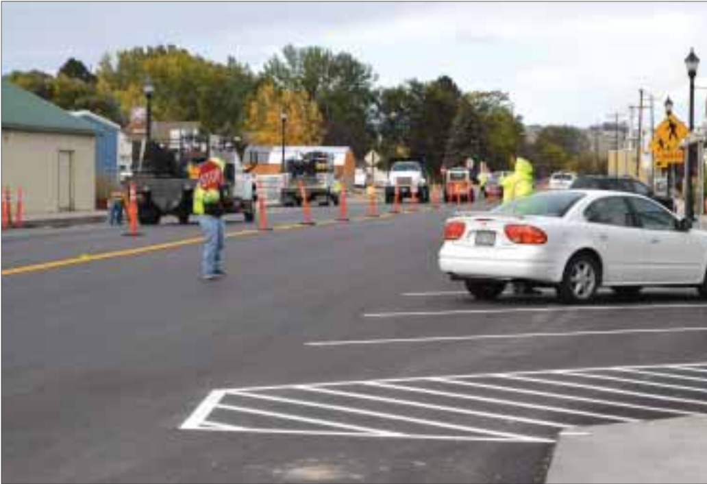
Flaggers stand on West Idaho Avenue west of 2 nd Street North on Monday as work continues on Homedale’s main thoroughfare. Parking stalls (and no parking areas) have been marked, and new signs posted to warn motorists of upcoming pedestrian crossings.
