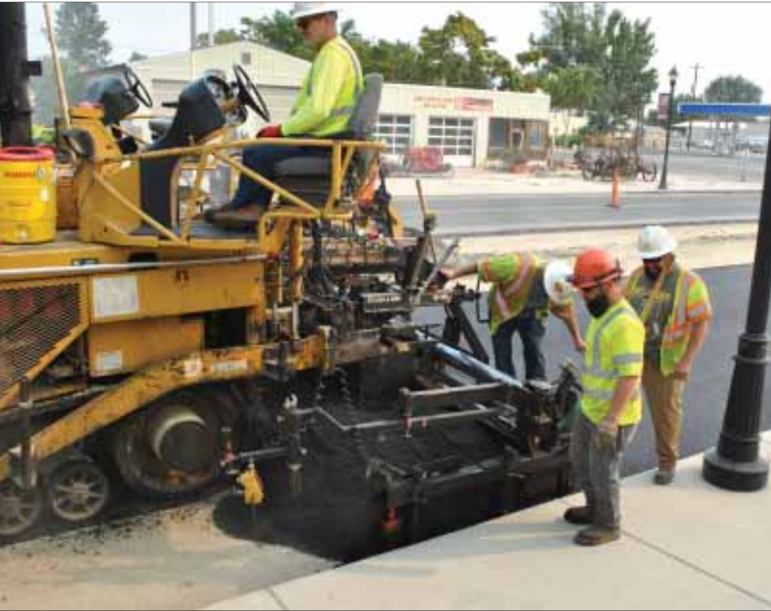
A Knife River Corp., crew lays down blacktop in front of the old Homedale Realty building on East Idaho Avenue on Monday on its way to completing Phase 3 of the Idaho Transportation Department project through the heart of Homedale. When work is finished on this stretch, crews will switch to the south side of West Idaho Avenue to finish up.
