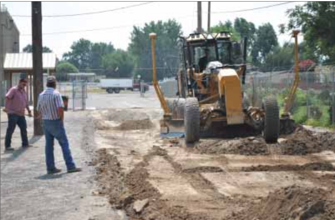
A Thueson Construction crew began excavation of the roadway along the west side of the Owyhee County Fairgrounds on Aug. 16.
