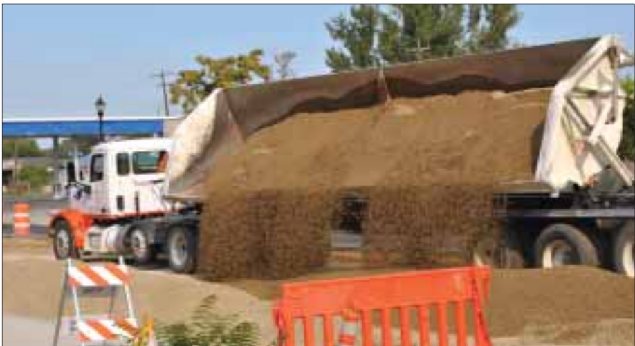
The delivery and compaction of dirt for the East Idaho Avenue roadbed in front of Bette Uda City Park began Monday.
