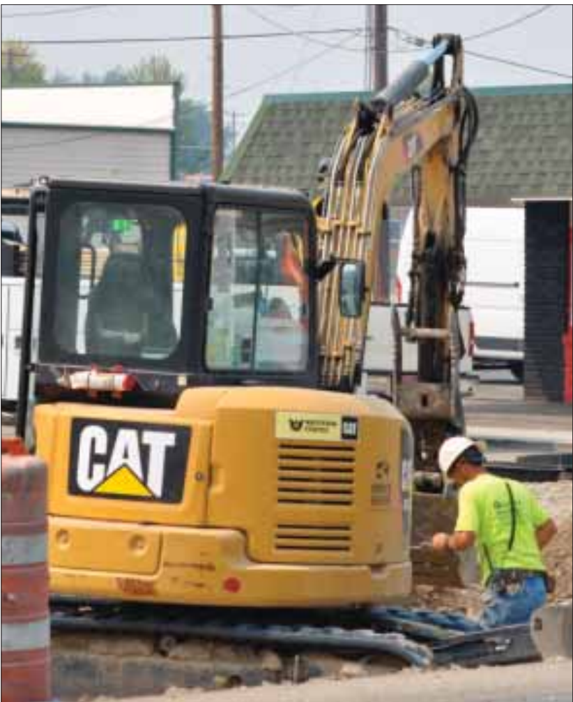
Roadway re-construction work continued last week on the south side of East Idaho Avenue in Homedale. Busy Knife River Corp. crews endured the seemingly endless hot summer days to continue their tasks. Once work is complete on this section of the highway, crews will move to the south side of West Idaho Avenue for the final phase of the project.
