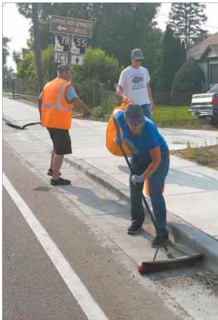
Marsing Beautification Project president Julie Franklin (right) puts a little elbow grease into her cleaning duties on Main Street in Marsing, while Robert Bell (left) and city engineer Kirby Cook lend a hand. The orange bags and orange safety vest were provided by the Idaho Transportation Department. Submitted photo
