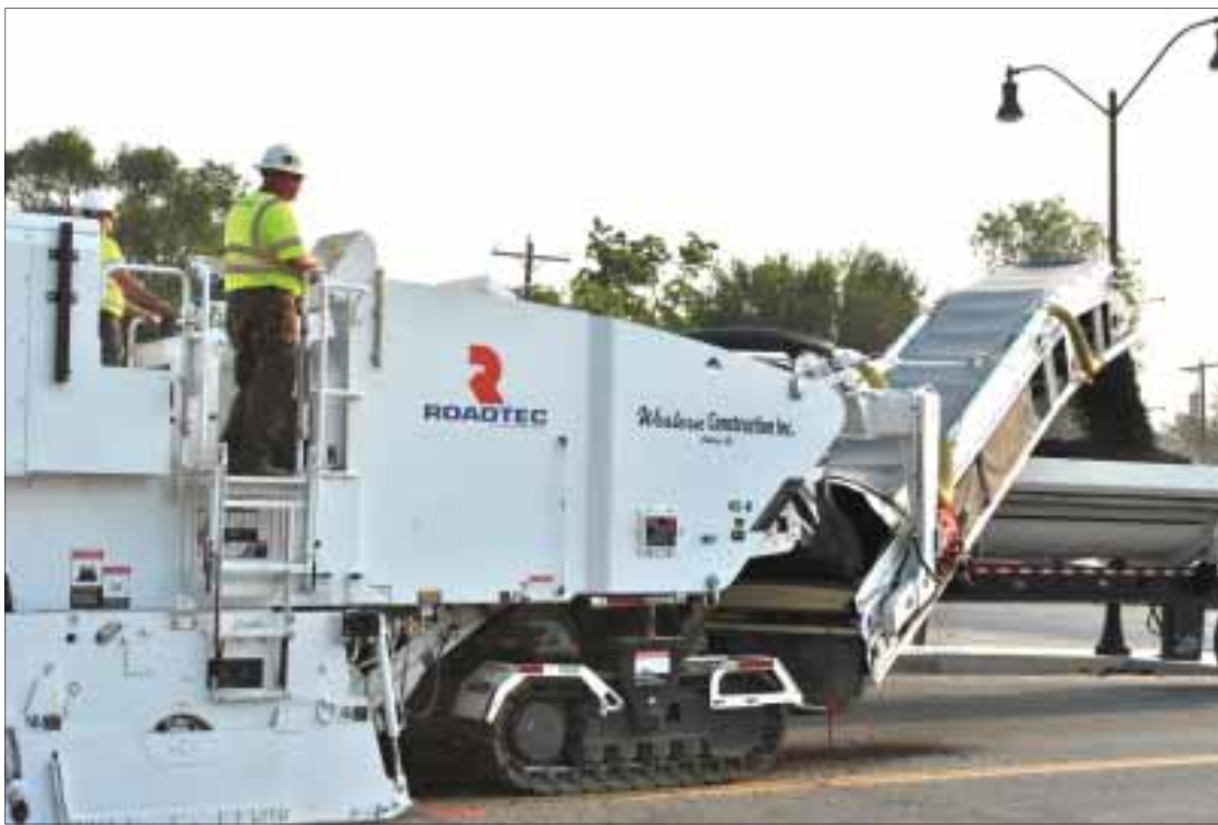
The destruction of the north side of East Idaho Avenue from Main Street to 4 th Street East was completed last week. Traffic has been moved to the south side of the street and barriers put up in front of some businesses in the first block of East Idaho.
