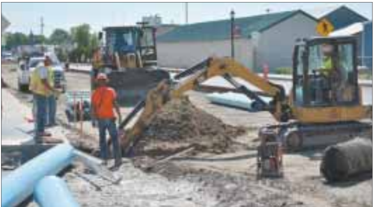
Trenchwork like this near the Homedale Senior Center will also be carried out on the east end of Idaho Avenue.
