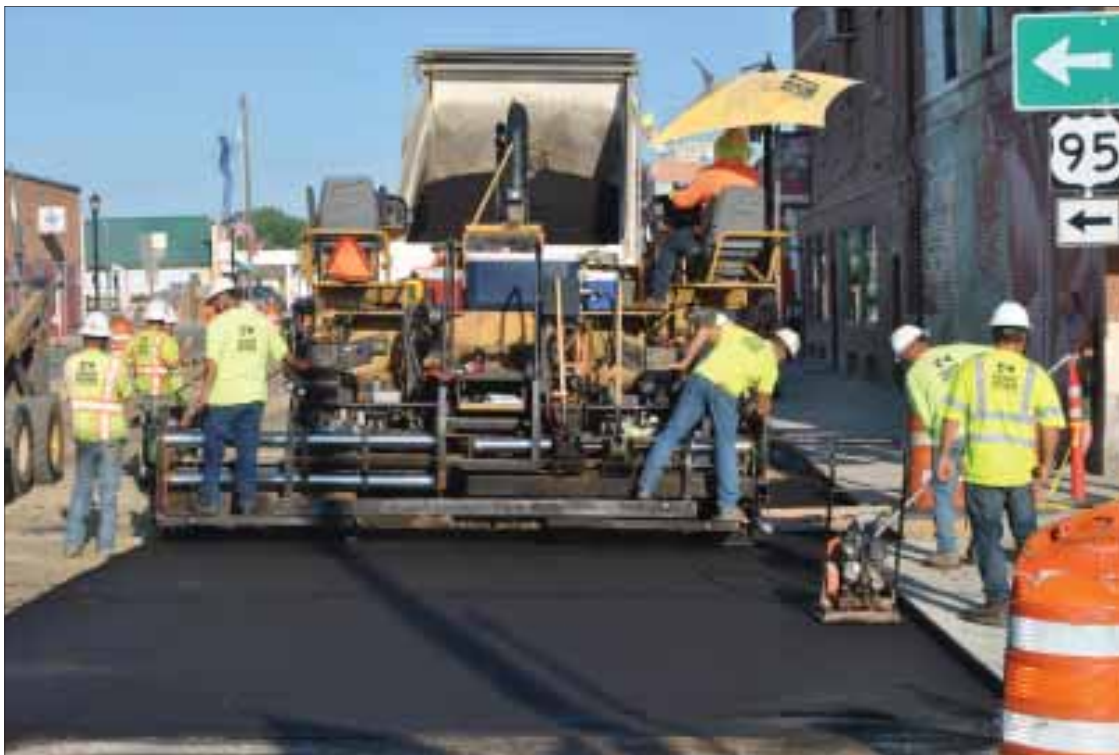
Above: Knife River Corp. started paving West Idaho Avenue from Main Street to 4 th Street West on Friday. Below: One Knife River crewmember followed the paver, testing for consistent depth of the freshly laid blacktop.
