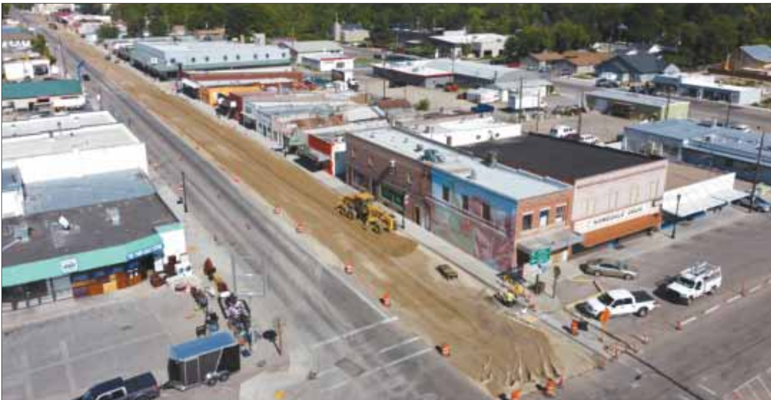
Knife River Corp., crewmembers work in a trench near the corner of West Idaho Avenue and North Main Street on Thursday in the midst of the massive reconstruction project for Homedale’s main thoroughfare. Photo by Jimmy Gross / Freedom Droneworks
