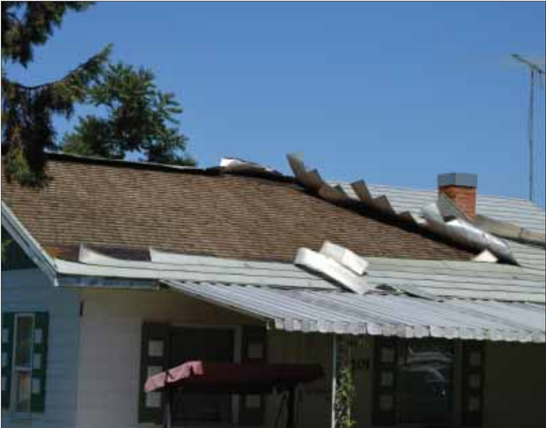
A house on the northeast corner of East Washington Avenue and North 1 st Street East received damage when the wind blew strips of metal roofing off, exposing a practically pristine shingled roof underneath.
