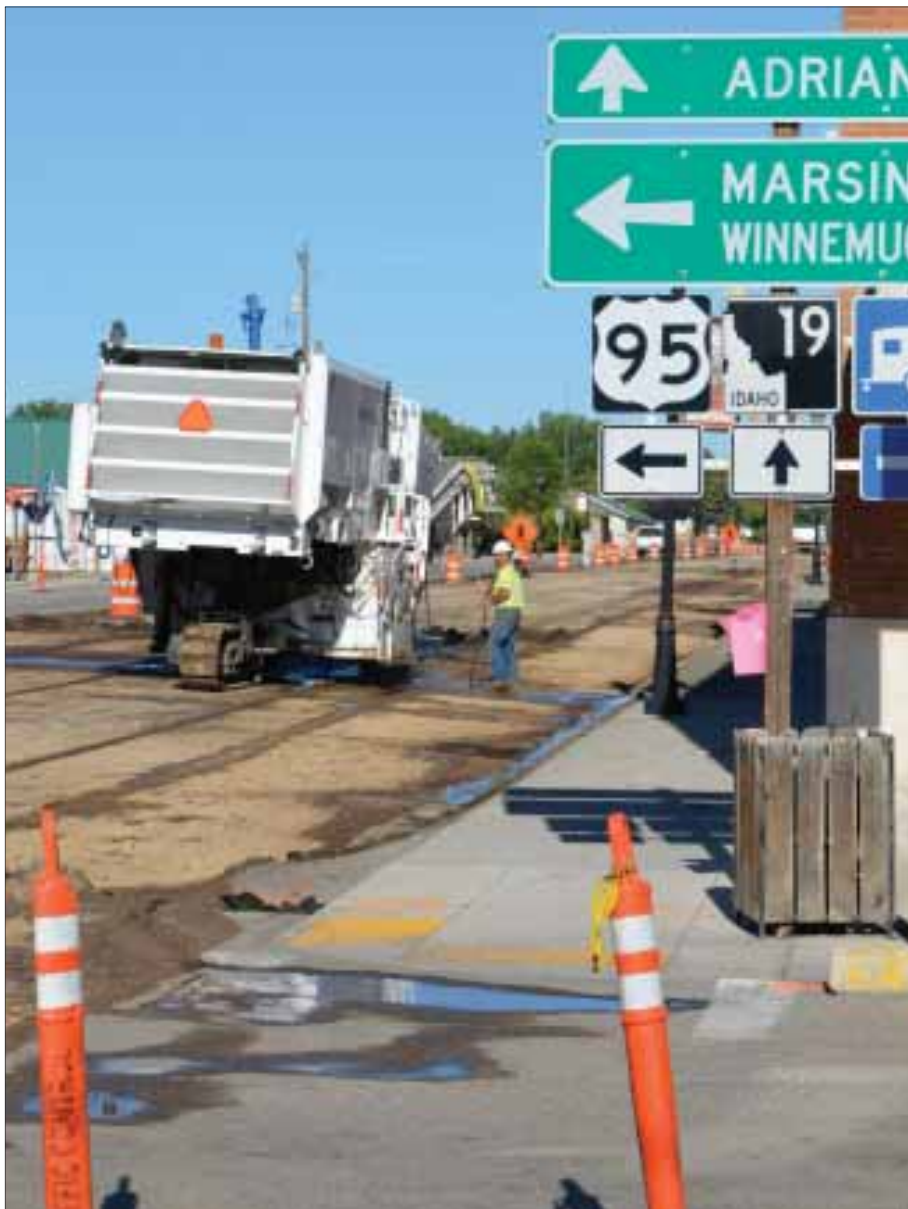
A Knife River Corp., construction worker cleans off an asphalt profiler on Thursday. The Idaho highway 19 rehabilitation project through Homedale began June 14, and the north side of Idaho Avenue from Main Street to 4 th Street West is torn up.
