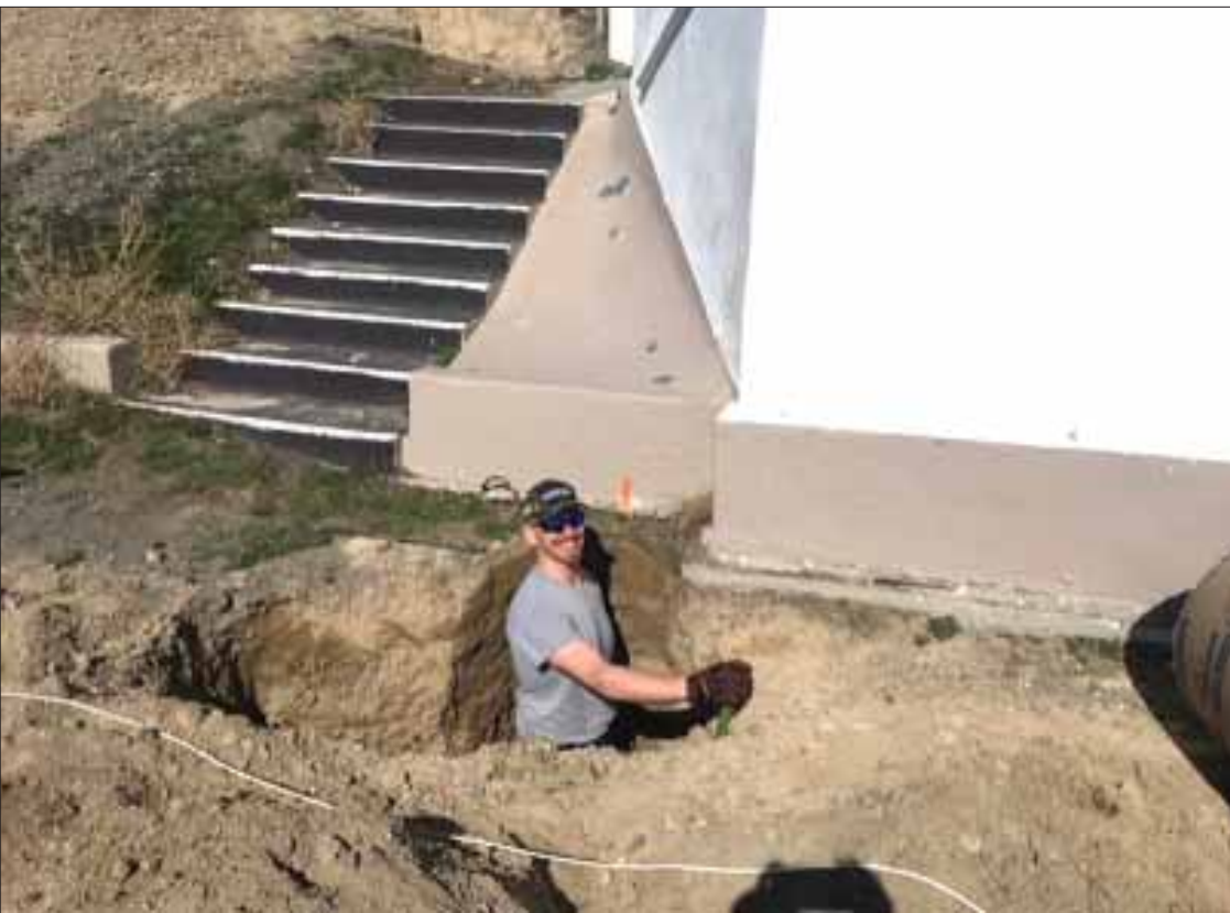
The project to put a permanent cover over the Lizard Butte Sunrise Service platform northeast of Marsing has included digging holes for footings (above) and placing posts and cross pieces with heavy equipment (below). Submitted photos
