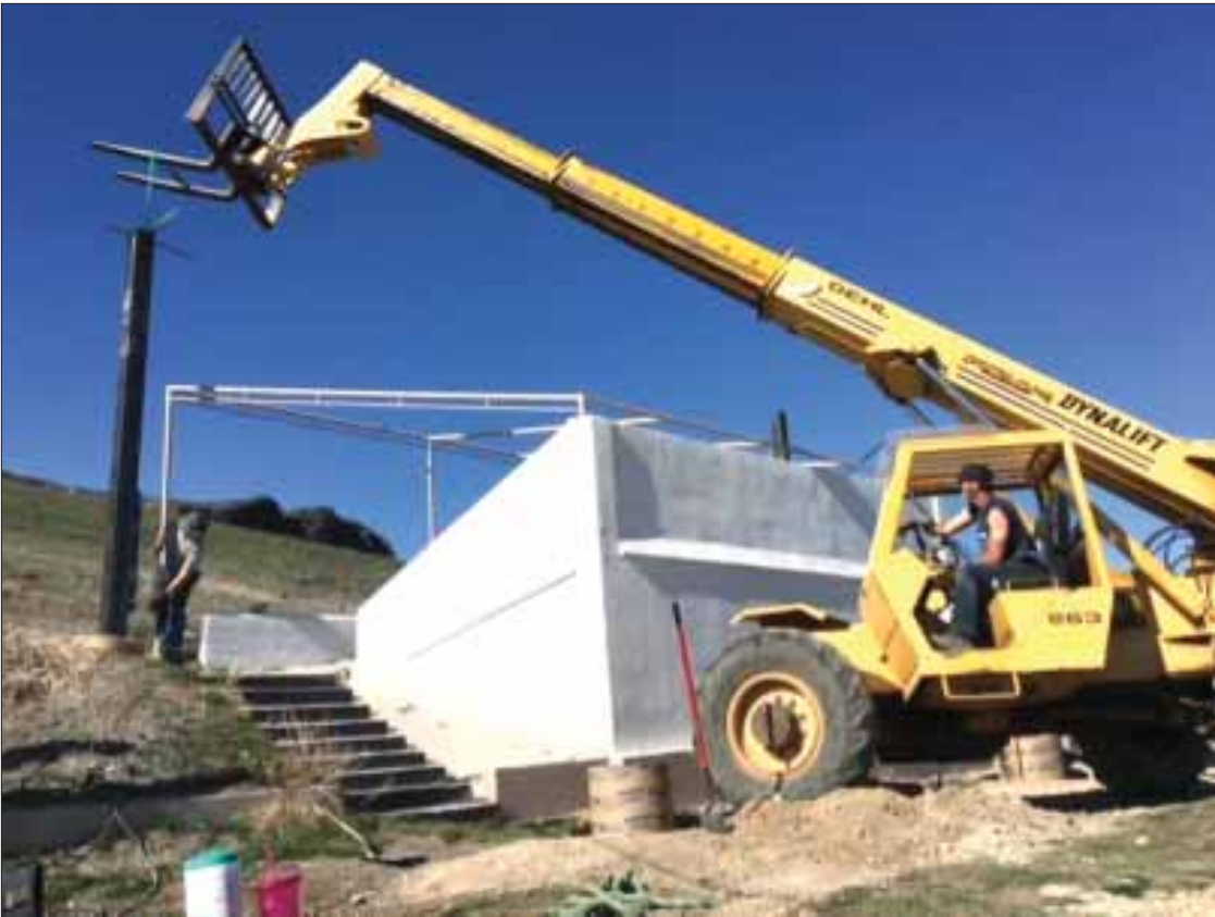
The project to put a permanent cover over the Lizard Butte Sunrise Service platform northeast of Marsing has included digging holes for footings (above) and placing posts and cross pieces with heavy equipment (below). Submitted photos
