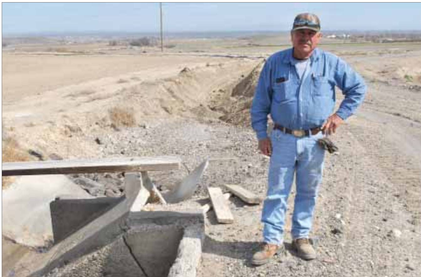
Servando Zalazar and his crew did some cleanup work on Thursday at Big Pump Ditch off Oregon highway 201, just past the state line.
