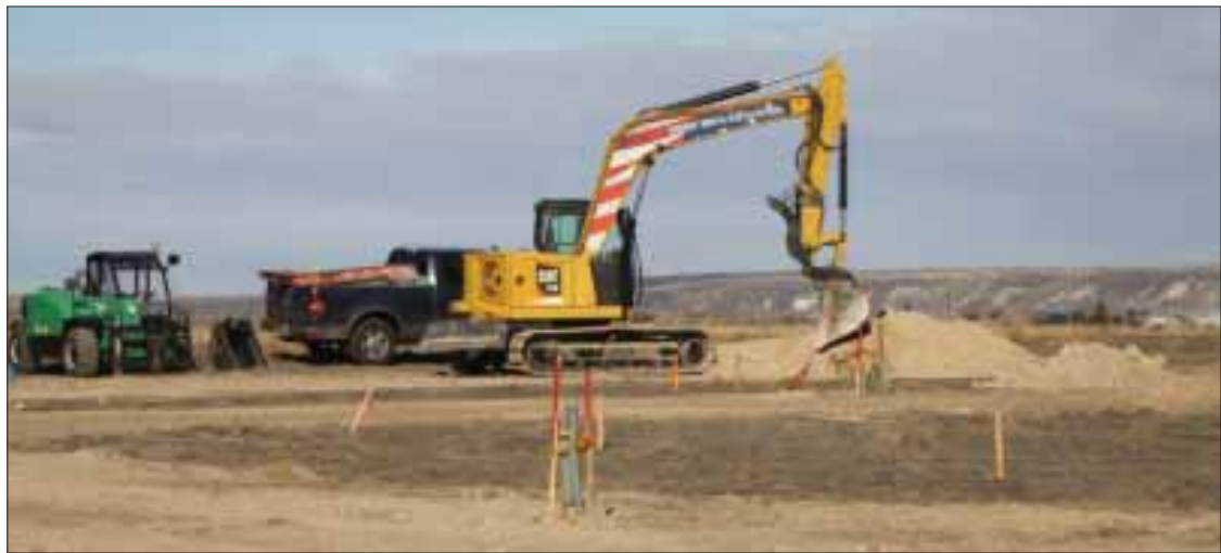
Crews have begun moving dirt as the first phase of construction gets underway on a new Bureau of Land Management Boise District wildland fire station in Bruneau. BLM photo
