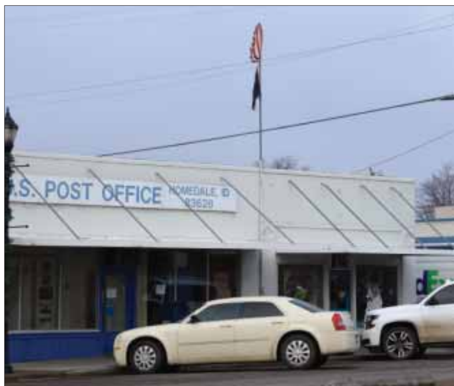
The U.S. Post Office in Homedale re-opened on Jan. 31, nearly four months after electrical and flooring work began.
