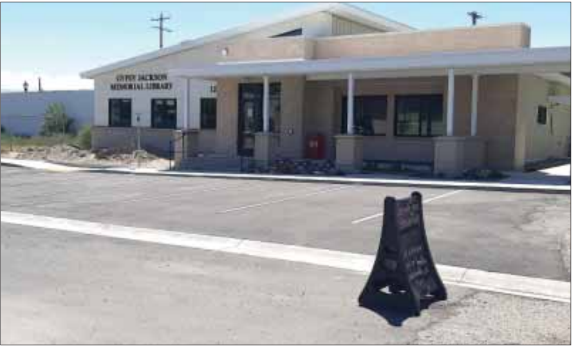
June — After a long-delayed opening, and two closures for mitigation of mistakes made during the construction process and COVID-19 concerns, Homedale’s Gypsy Jackson Memorial Library was back in business for good.
