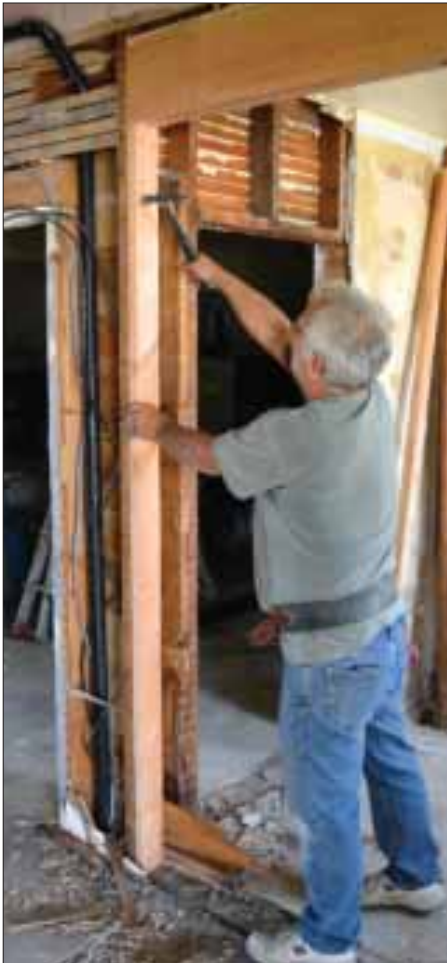
May — General contractor HCD, Inc. began remodel work on the new Marsing City Hall, which would be housed in the old Sandbar Restaurant with a Cause. Work was completed in July.
