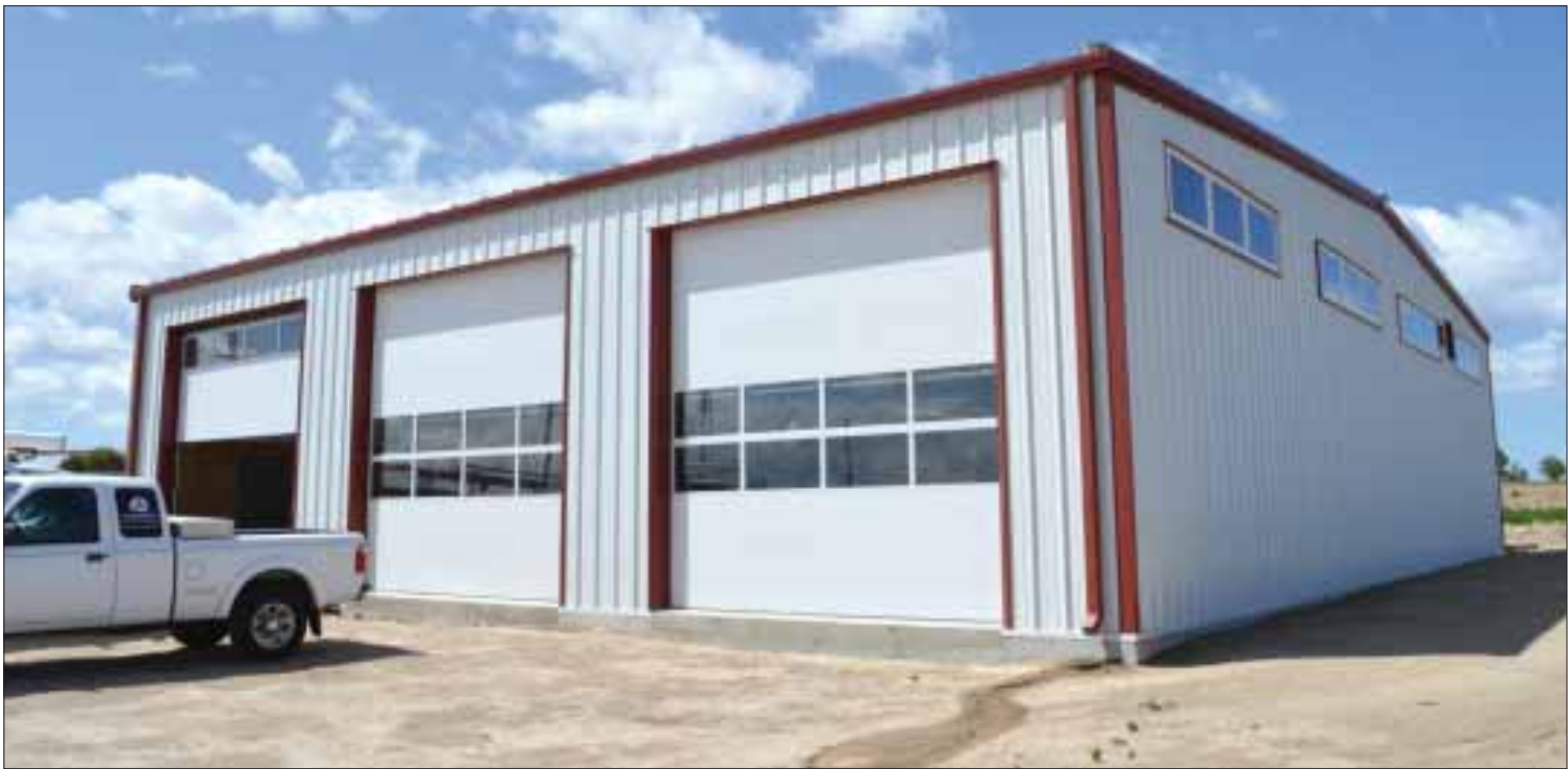
June — Construction of the Marsing Rural Fire District’s substation on Walker Lake Road in Canyon County was completed.
