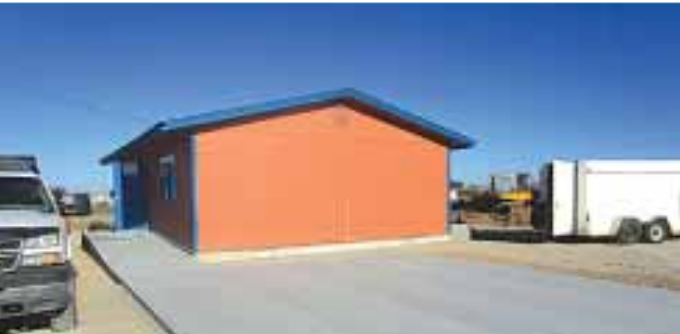
Work continues on the county's Grand View substation — both inside and out. Submitted photos
