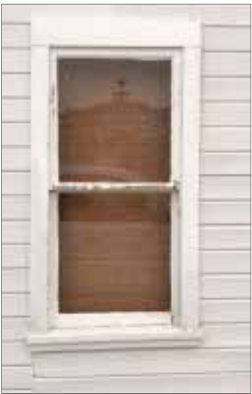
The Our Lady of Queen of Heaven Catholic Church is reflected in one of the Oreana Community Hall windows that volunteers are working to replace. Submitted photo
