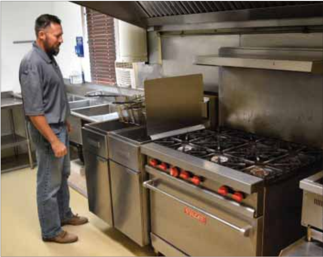
Marsing city code enforcement officer Cory Callison examines the stove and fryers in City Hall’s kitchen. Metro Meals on Wheels will use the kitchen to provide congregate meals on Mondays, Wednesdays and Fridays beginning next week.
