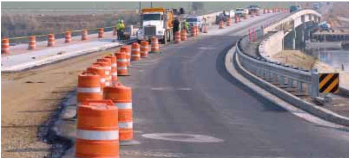
Work was nearly complete on Friday on the Snake River bridge in Marsing. Wadsworth Brothers crews still needed to complete some north side paving including part of the bridge deck and the new Island Park access ramp.
