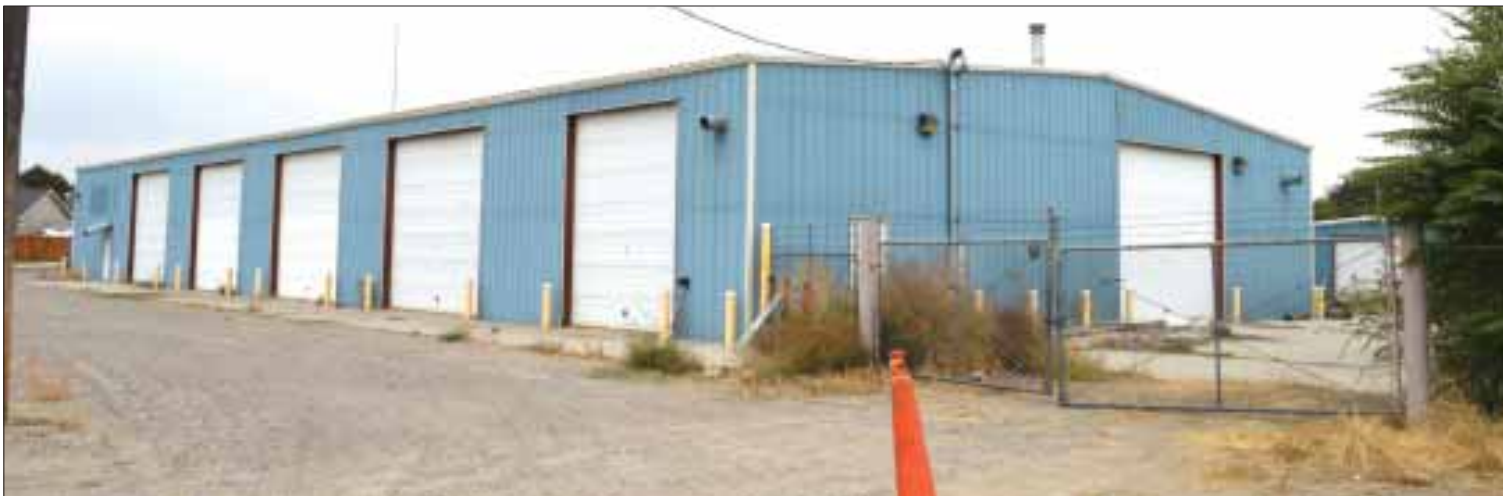
There is room on the west end of the main building to hold board of directors meetings, South Board of Control manager John Eells said of the new 10,000-square-foot repair shop site.
