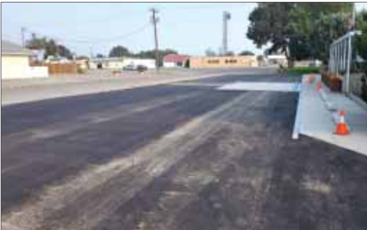
Building on Christian Sharek’s Eagle Scout project, blacktop was recently added to the Eastern Owyhee County Library’s parking lot. Photo by Mandi Boren
