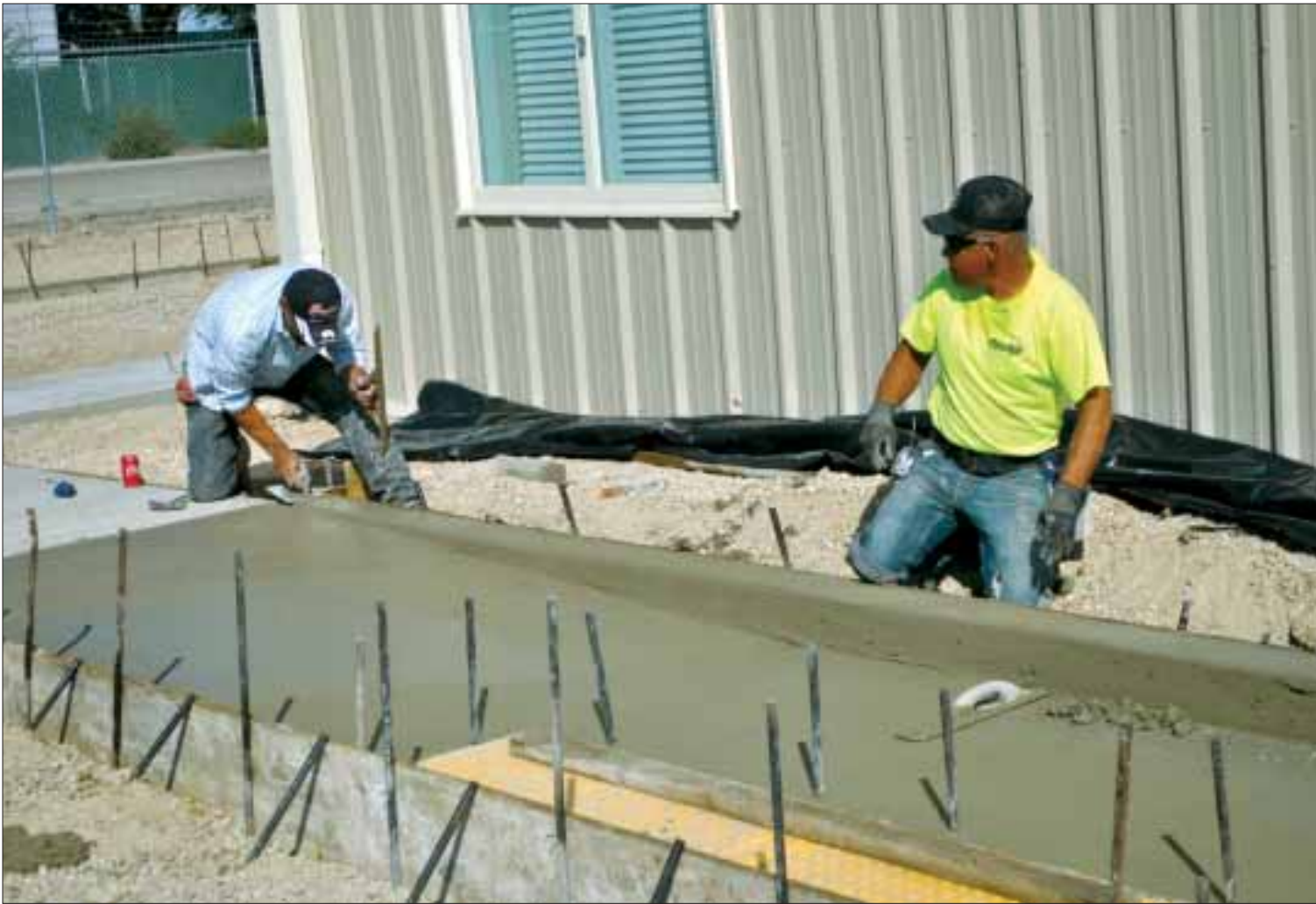
Manuel Rangel V (left) and Alfonso Cisneros of Pusher Construction work on the new sidewalk in front of the Owyhee County Community Center in Homedale on Thursday. The sidewalk is part of a larger project to put in a new parking lot.
