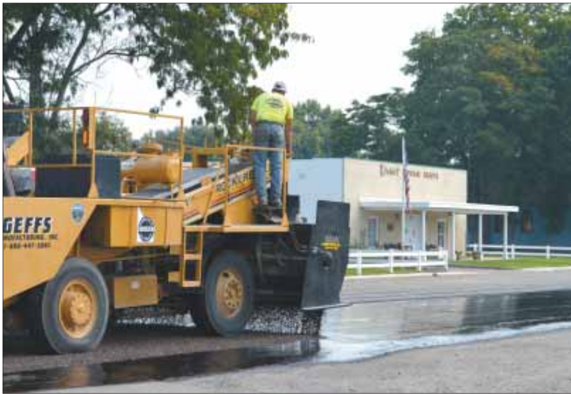
The Homedale Highway District maintenance crew, including Director of Highways Dan Herman, manned a machine to lay rock chips down on East Owyhee Avenue recently in a joint City of Homedale-HHD project.
